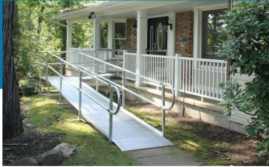
Installation of Ramps
