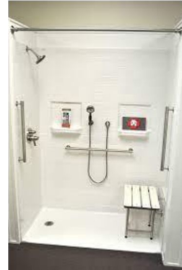
Modifications to bathroom
